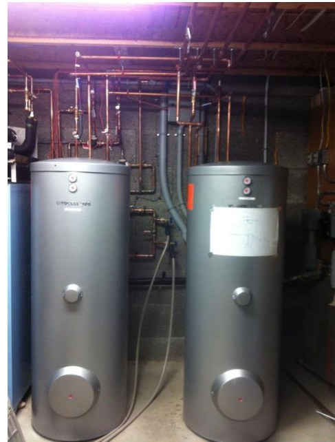
Fig. 4.10 Heat rejection circuit (before insulating)
