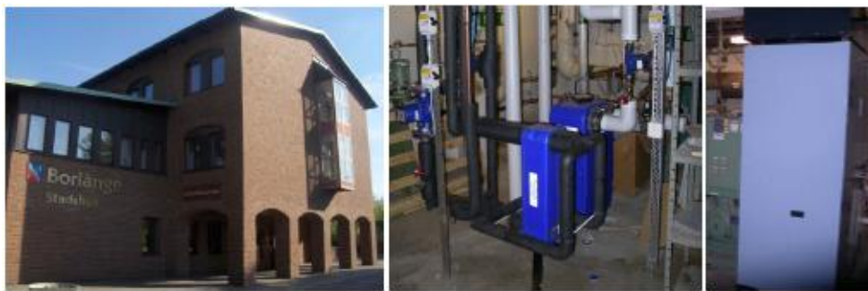
Figure A.2 Installation of Climatewell® version 7.0 chiller in Project-1 (Nurenz, 2010)
