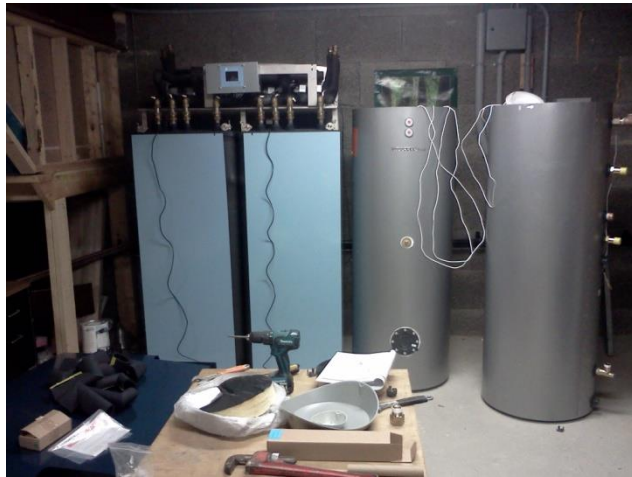
Fig. 4.10 Heat rejection circuit (before insulating)
