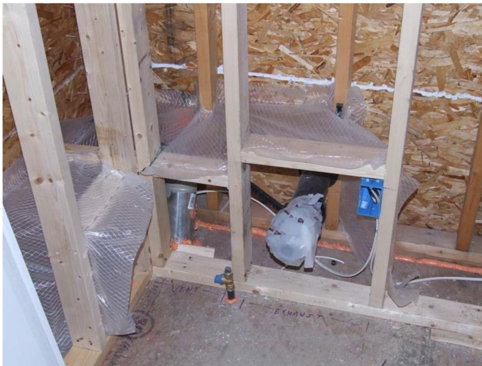
Figure 7: DWS blocking off penetrations (Aldrich, Arena, & Zoeller, 2010).
