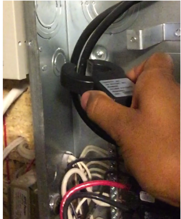
Figure 3: Induction clamp installation
