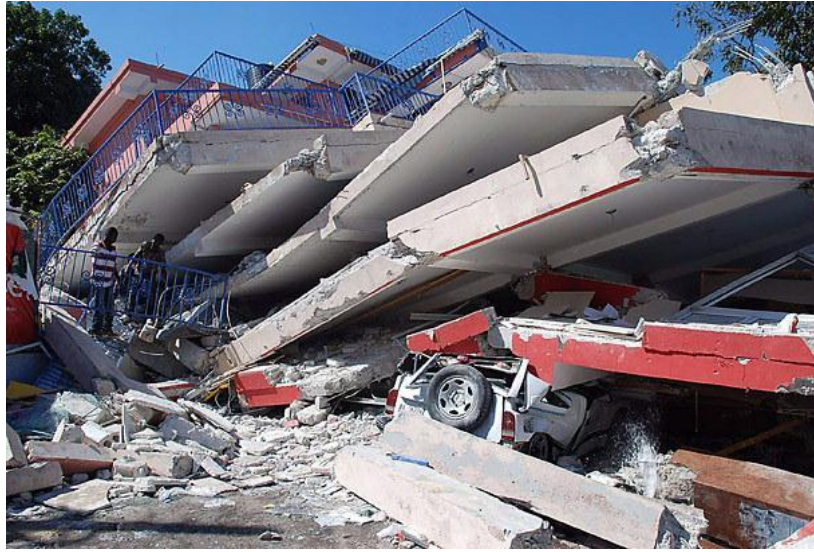
Figure 2-2 Pancake style building collapse
