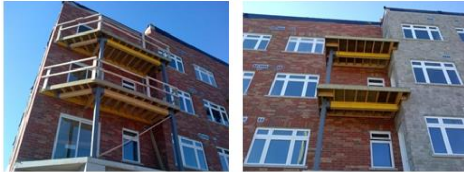
Figure 9: Thermally Broken and Structurally Separated Balconies from the Building Structure located in Fergus, Ontario
