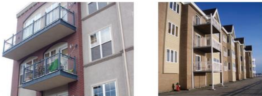
Figure 8: Left: Balcony Precast Unit with Threaded Rods. Right: Stand-alone Supporting Structure [21]
