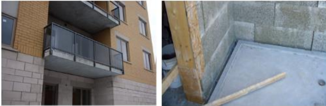
Figure 7: Balcony offset Point Supports Precast Balcony Supported Intermittently to Break Thermal Bridge [21]
