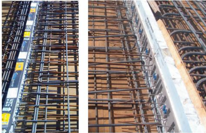
Figure 11: Installed Schöck Isokorb® Thermal Break in Canadian Building's Balconies [22]
