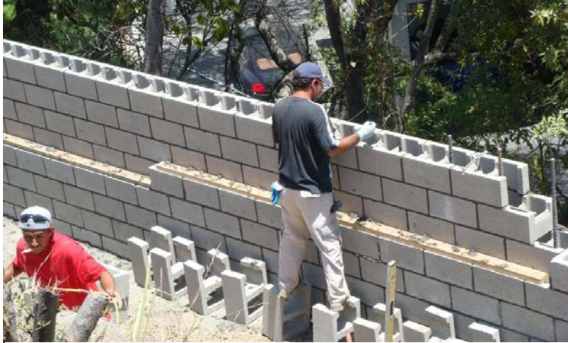
1.6 - Concrete Masonry Unit (CMU) Wall - Image Retrieved from http://www.mikepearsonconstruction.com/wp-content/uploads/2012/05/DSC00155-1.jpg
