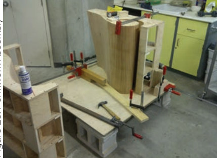
Figure 28: Formwork Assembly
