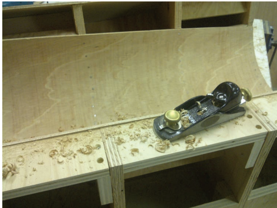
Figure 07: Heavy-Light Concrete Texture Detail Figure 08: Heavy-Light Fissure Detail Figure 09: Heavy-Light Hand Planing Formwork
