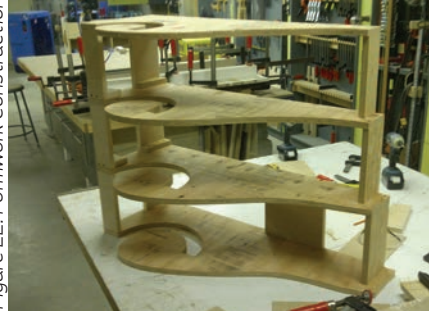
Figure 22: Formwork Construction
