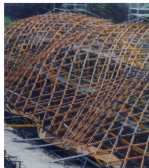
Figure group 7.4. Formation of the Downland gridshell. Edward Cullinan Architects, 2002
