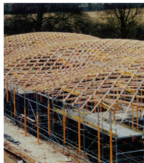
Figure group 7.4. Formation of the Downland gridshell. Edward Cullinan Architects, 2002
