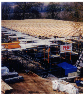
Figure group 7.4. Formation of the Downland gridshell. Edward Cullinan Architects, 2002
