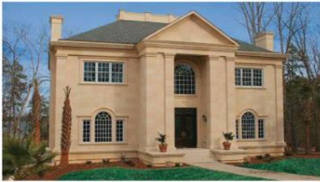
EIFS Applied on a Low-rise Residential Building in Lexington, South Carolina.
