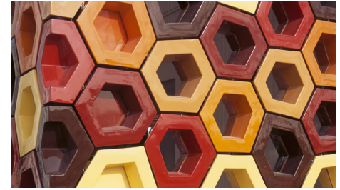
Figure 46: This cladding for the World Expo 2005 Spanish Pavilion by FOA aims to reflect the colours of Spain and takes cues from both Christian and Islamic traditions. The hexagonal tiles vary in shape, colour and arrangement.
