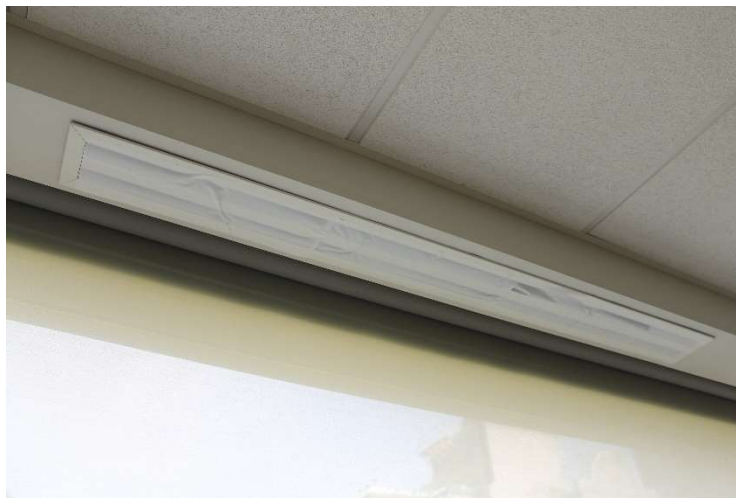
Figure 12. Occupants taped supply vent shut due to cold air.
