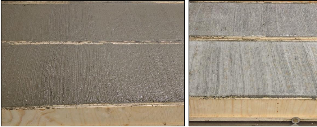
Figure 3-30: Surface Preparation of Large Slabs
