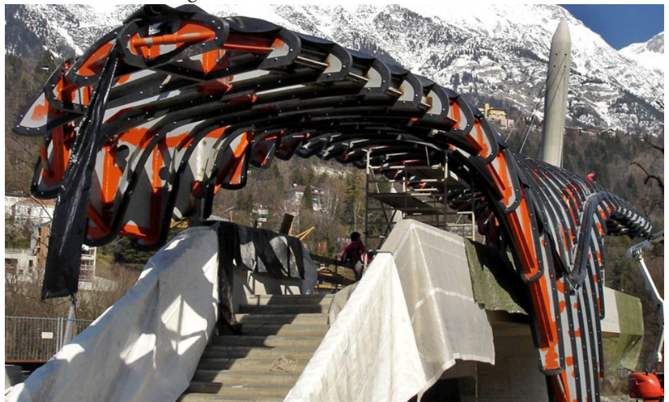
Figure 10: One of Zaha Hadid's Nordpark stations under construction, showing the unique plates and their associated gaskets.
