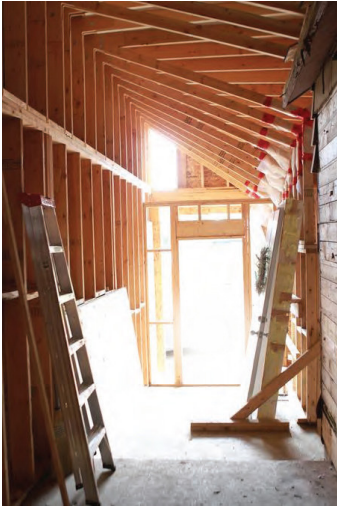
Figure 24: The interior hallway, showing the sloping rafters associated with the rise in the floor.
