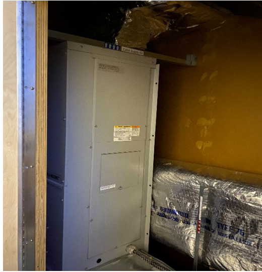
Figure 7.0: AC unit placed at the back of the Cabin.
