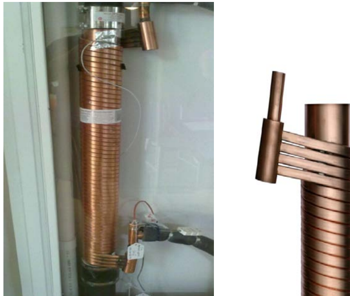
Figure 6-2: Overview of PowerPipe R3-36 unit in House-B and the wrapped tubes view
