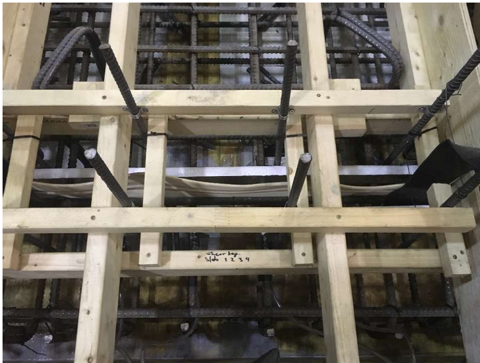
Figure 3-11: The integration of membranes into the formwork & details of installation of dowels
