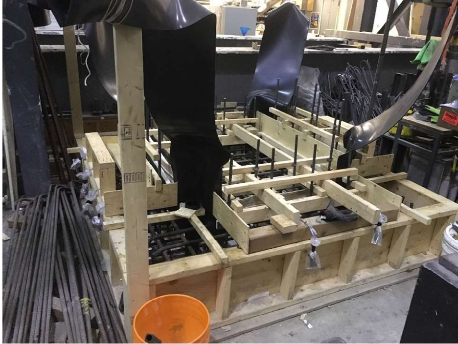
Figure 3-10: Installation of neoprene membranes using the posts and the template
