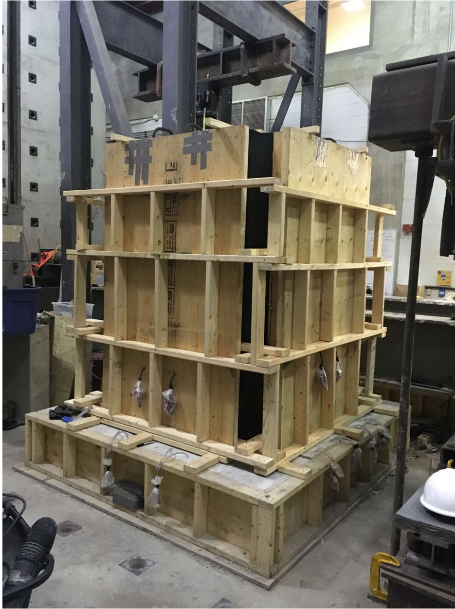
Figure 3-20: The closed formwork with the bracing before the concrete pouring.
