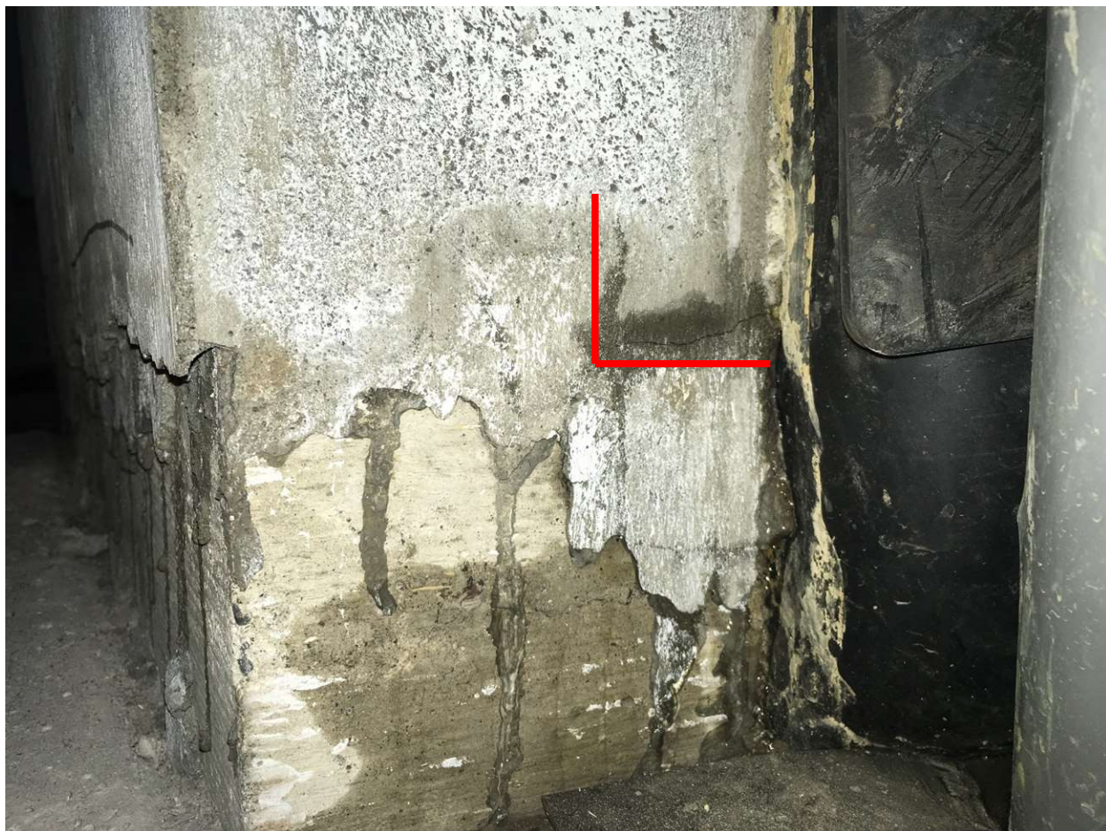
Figure 4-58: Formation of cracks on the outline of the shear key in the US joint
