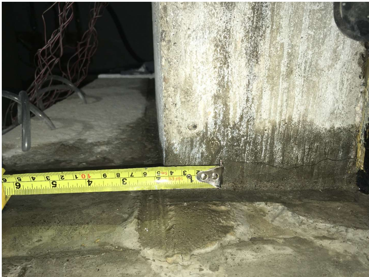
Figure 4-73: Formation of cracks along the joint between the wall and the base slab
