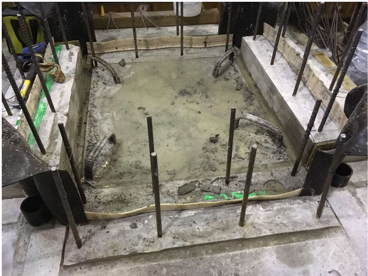
Figure 3-13: The fully built base slab after formwork removal
