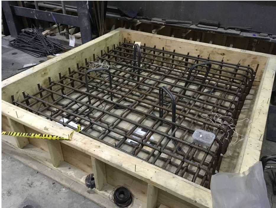
Figure 3-6: Installation of top reinforcements
