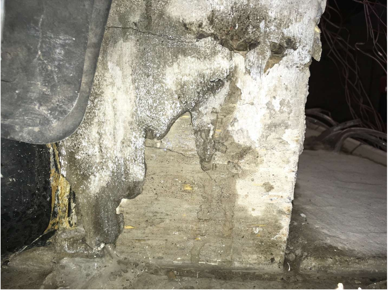
Figure 4-66: Formation of cracks along the construction joint.
