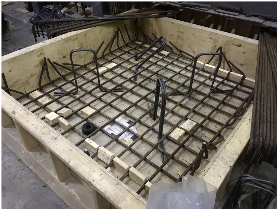
Figure 3-5: Installation of bottom reinforcements and crane handles
