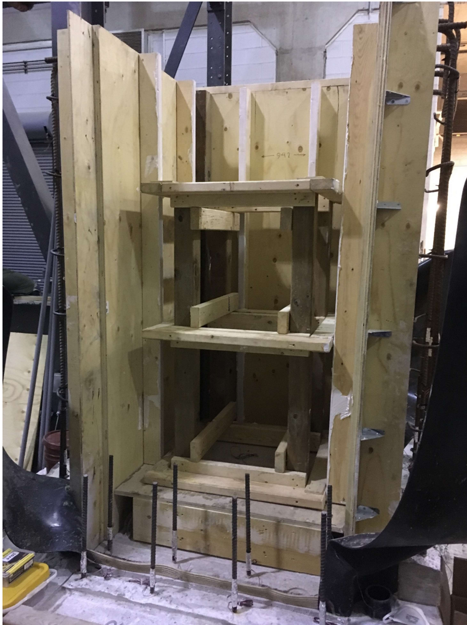
Figure 3-16: The inner formworks of the walls placed around the inner core
