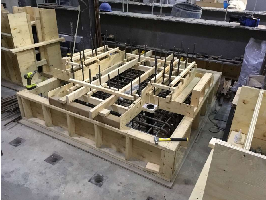
Figure 3-9: The template used for the formwork of the upturn parts
