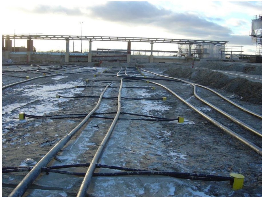
Figure 6 – Installation of vertical boreholes, UOIT, Courtesy of Groundheat Solar Wind [4]
