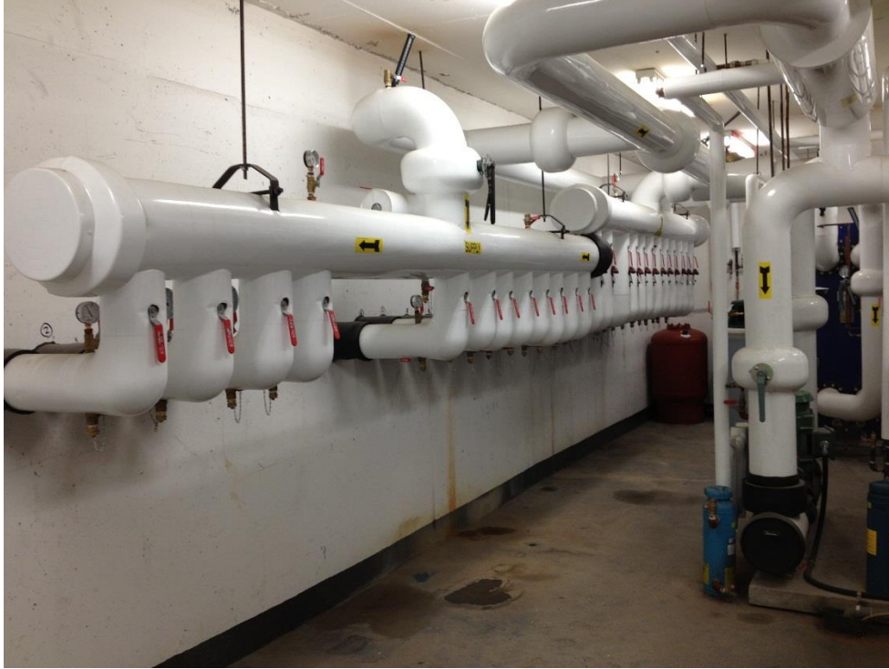
Figure 16 – Typical Supply and Return Manifolds (along wall), (courtesy of [4])
