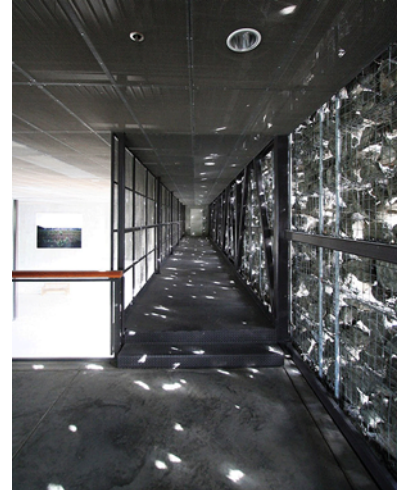
Fig 8.9 and Fig 8.10. Dominus Winery using basalt rocks for gabions, Herzog and de Meuron
