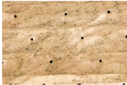
Fig 7.6 and Fig 7.7. Remnants of the tie bolts through which light filters into the dark of the inside space
