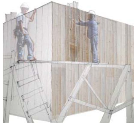
Birch shuttering for solid concrete walls
