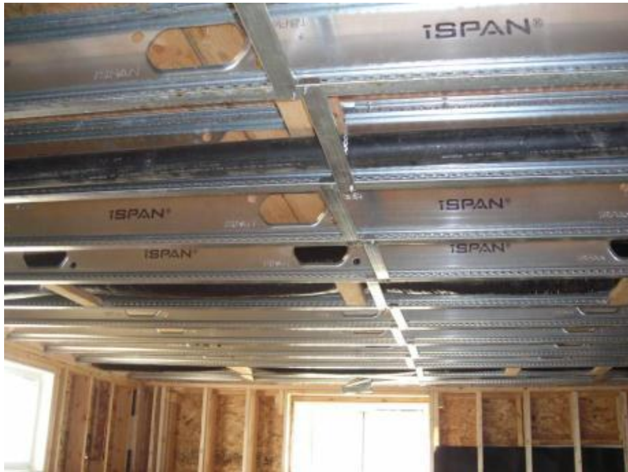
Figure 3.48: View of the bracing attached to the bottom flange of the joist in test site 1
