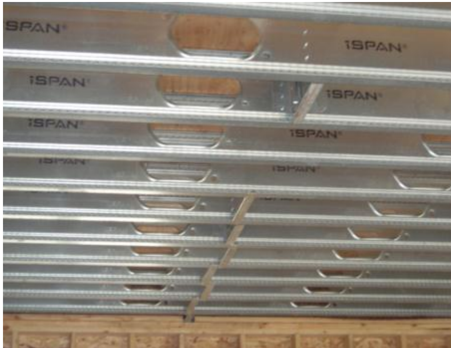
Figure 6.1: View of a typical floor built with iSPAN joists with edge-stiffened web holes
