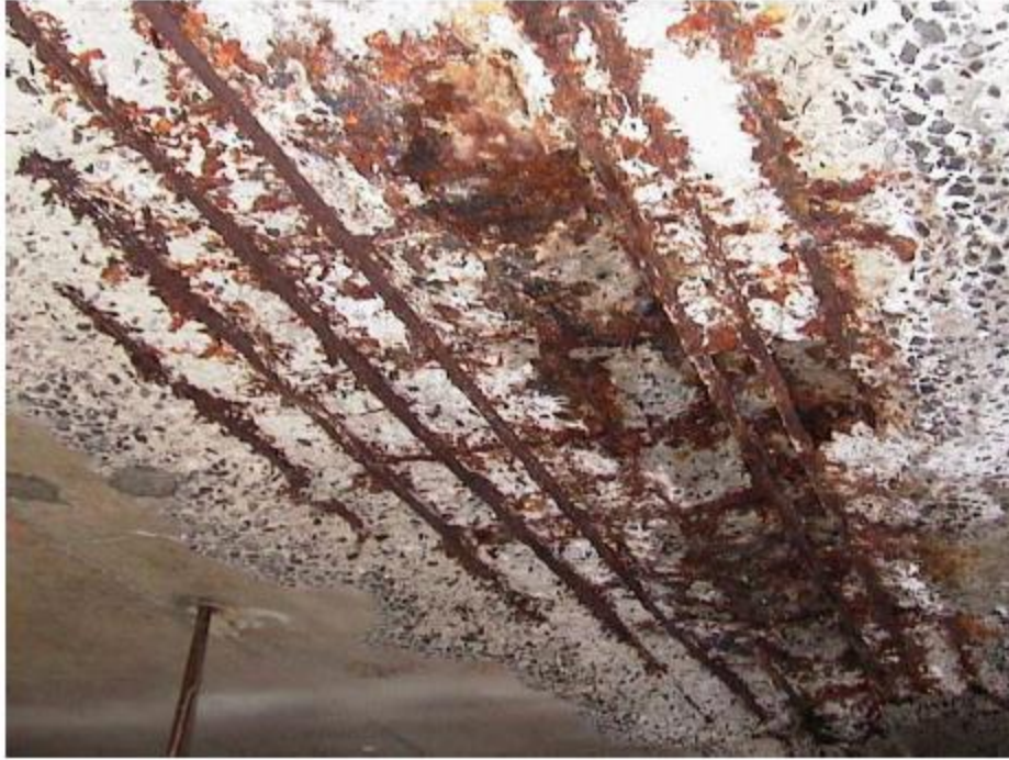
Figure 2.18 Corrosion of steel reinforcement in concrete Structures (Xiaoming et al., 2010)
