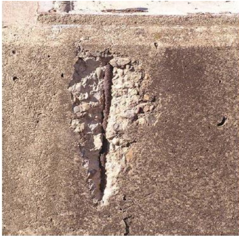
Figure 2.16 Corrosion and spalling induced by carbonation (Xiaoming et al. 2010)
