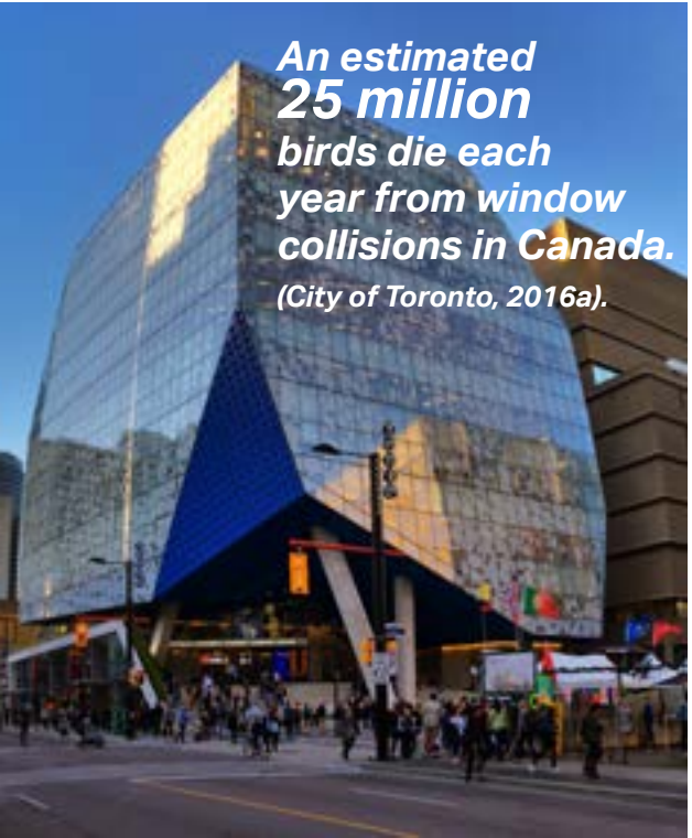
Figure 4 - This example of bird-friendly design is found downtown at the Ryerson Student Learning Centre. Visual markers are incorporated into the exterior glass which protects birds from colliding.
