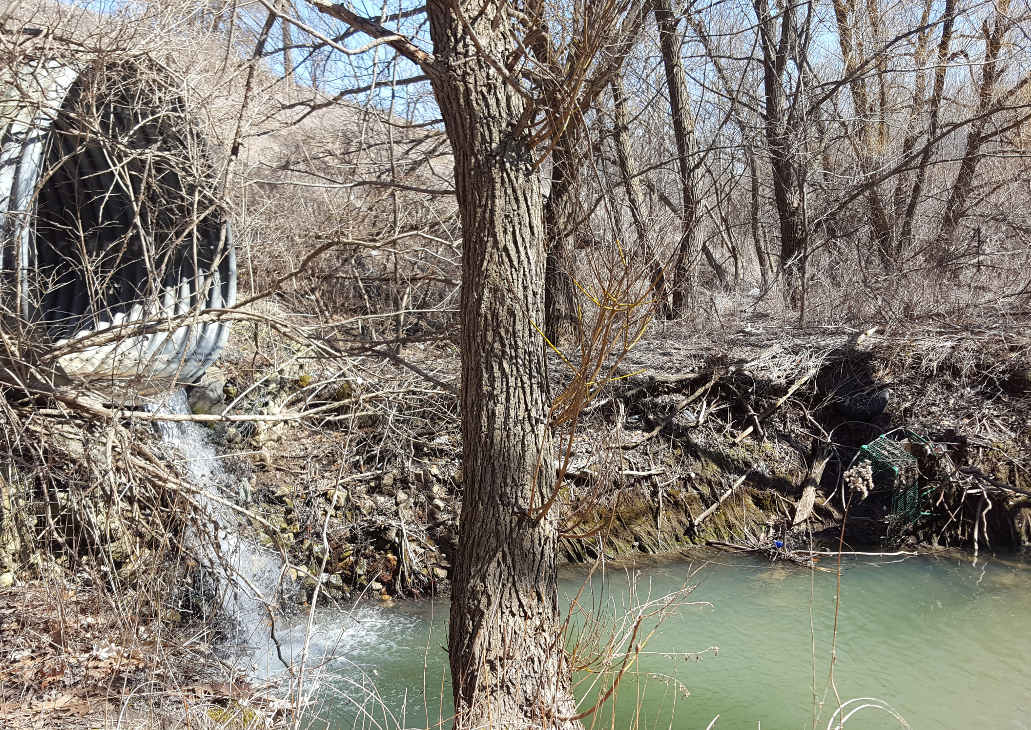
A pipe culvert connecting the water from Ellesmere Ravine across Ellesmere Road (2017, V. Racine)
