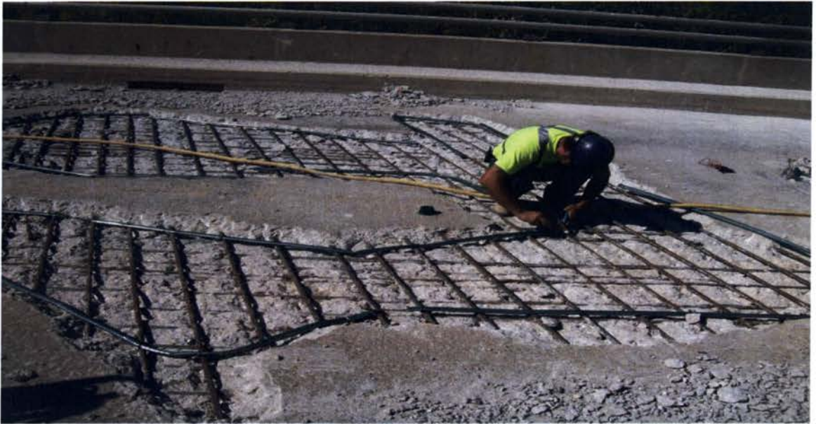
Fig.5.10 –installation of Zincribbon for bridge deck
