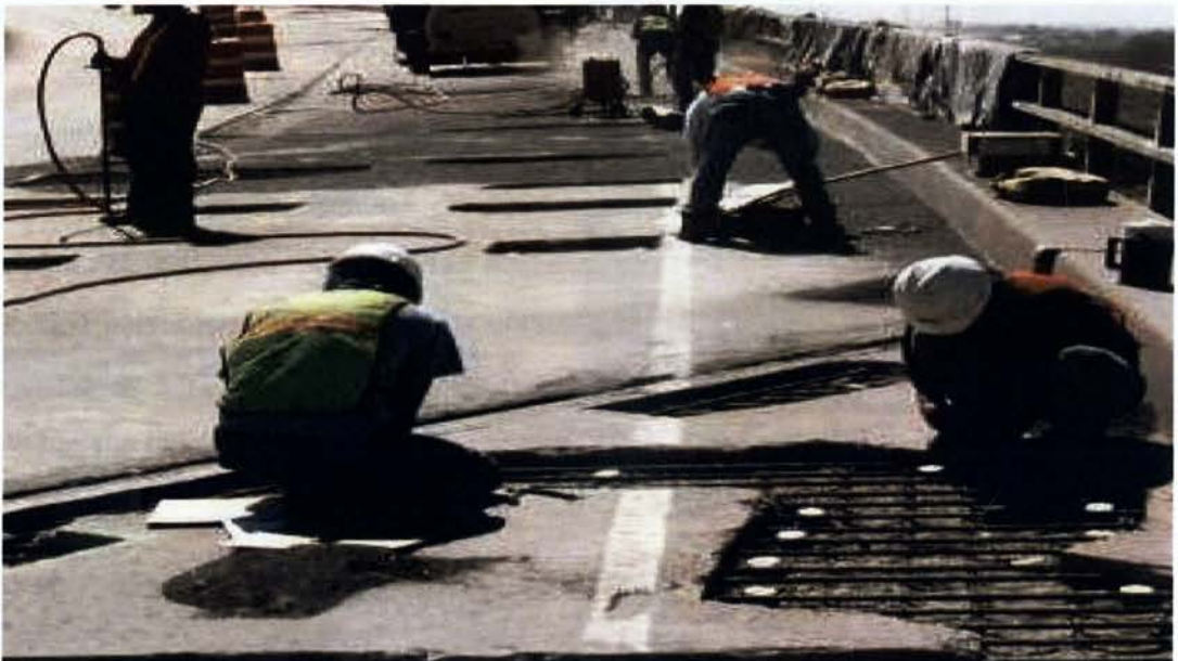
Fig.5.8 –installation of Embedded Galvanic Anode for bridge deck, Colorado
