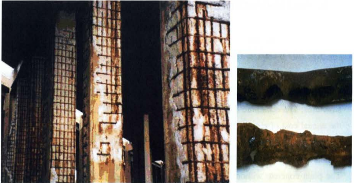
Fig.5.1 –Corrosion Ravaged Columns - Chicago, Illinois
