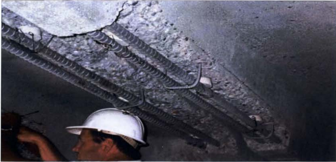
Fig.5.9 –installation of Embedded Galvanic Anode for beam
