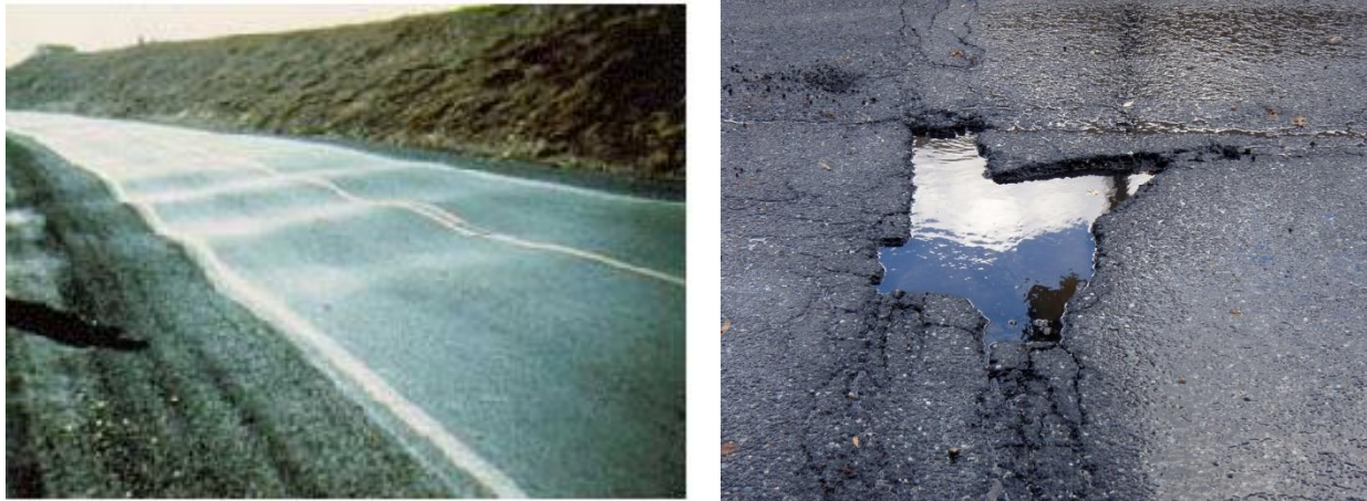
Figure 2-9 Waves and potholes in a pavement caused by frost action (Source: HTTP://WWW.FHWA.DOT.GOV ; HTTP://WWW.POTHOLE.INFO )
