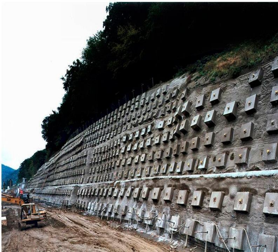
Figure 2-1 Soil nail wall (Source: HTTPS://SEMINARLINKS.BLOGSPOT.CA )
