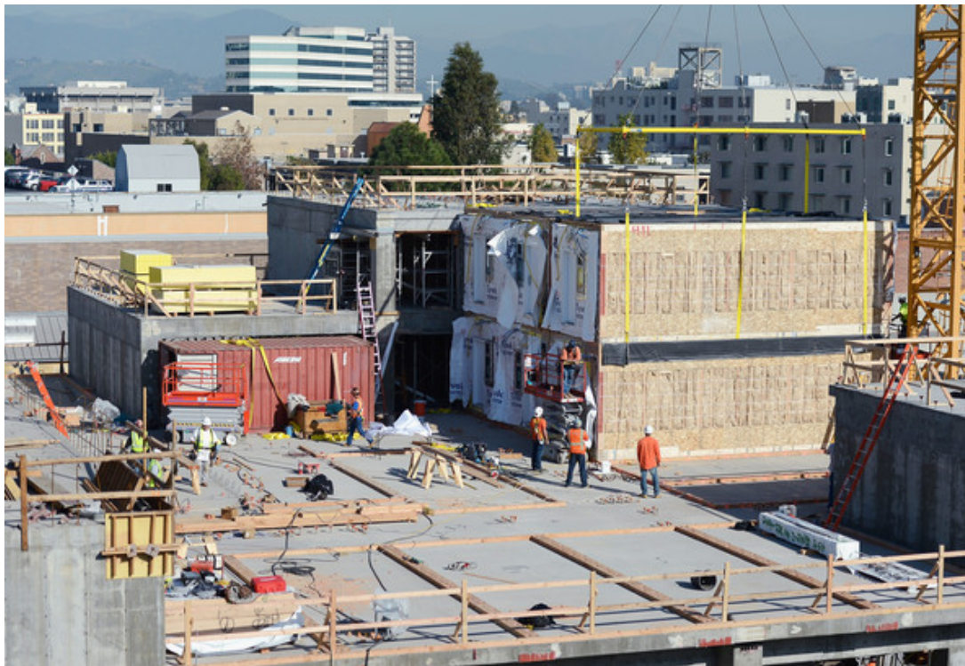
Figure 39: Star Apartments: Prefabricated residential units lifted into position. (Maltzan, M. 2013).
