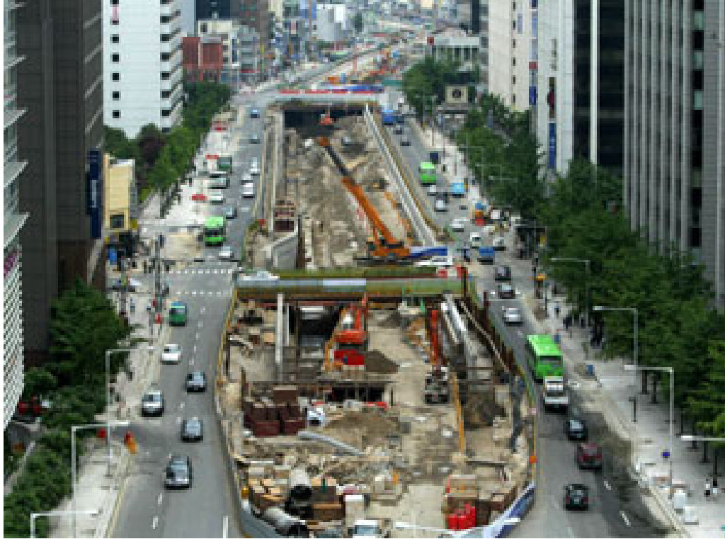
Figure 8: Removal of the elevated highway and dewatering the Cheonggyecheon Stream during reconstruction 2 .
