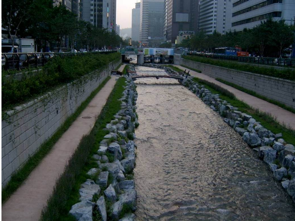
Figure 10: Photo taken upstream of Figure 11, applying armor stones along the banks 2 .
