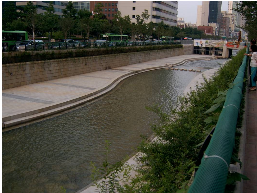
Figure 9: Meanders created by concrete banks in Cheonggyecheon Stream after the completion of the restoration 2 .
