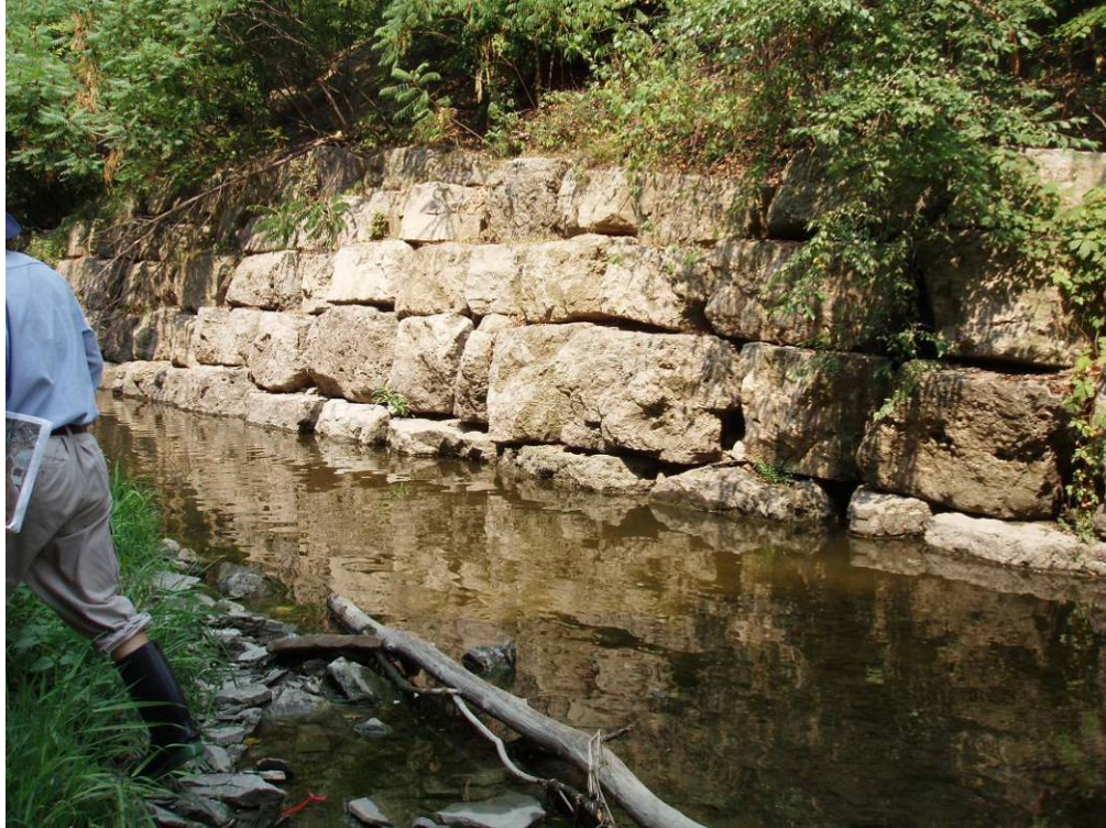
Figure 1: Structure applied in the late 1980's to straighten a section of the natural stream in Mississauga, Ontario, Canada.
