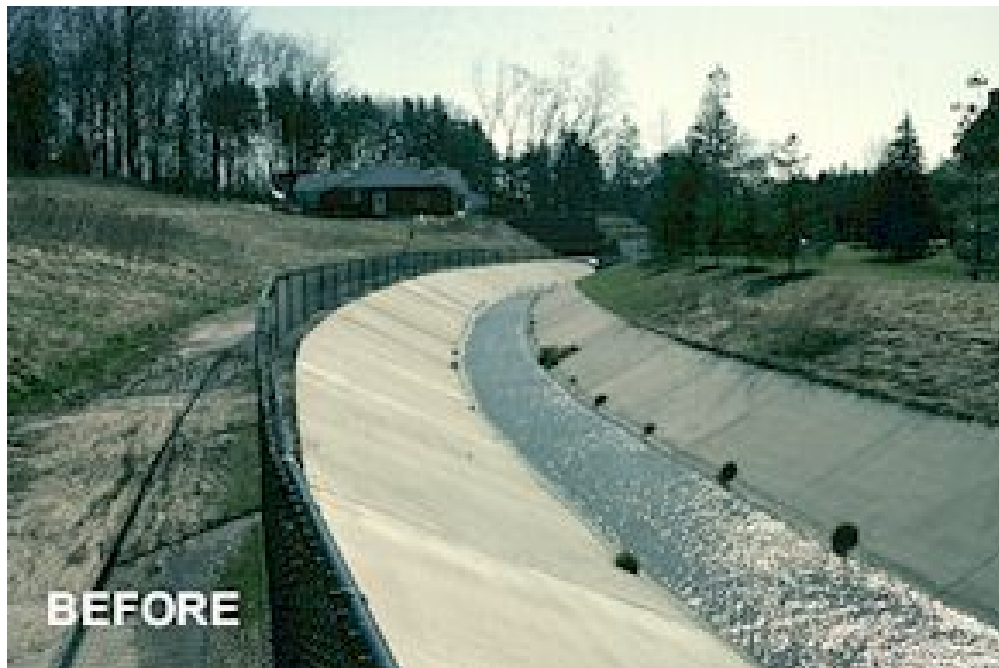
Figure 3: Concrete trapezoidal channel in Colonial Creek, Waterloo, Ontario, Canada before the restoration project (Harrington, 2003).
