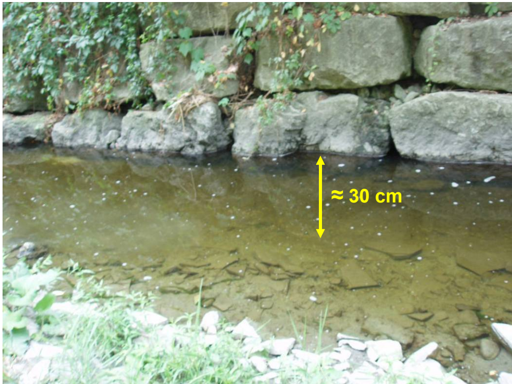
Figure 2: Close-up on Figure 1. Structure is severely undermined due to erosion problems and will likely collapse in the future.
