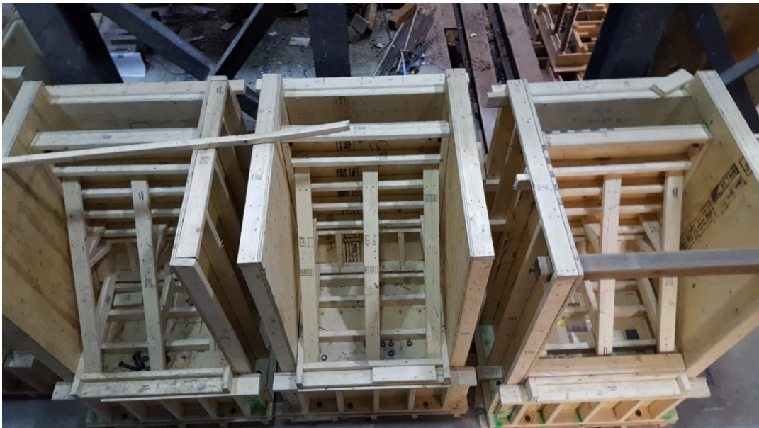
Figure 4.8: Typical formwork construction for TL-5 barriers in phase 2
