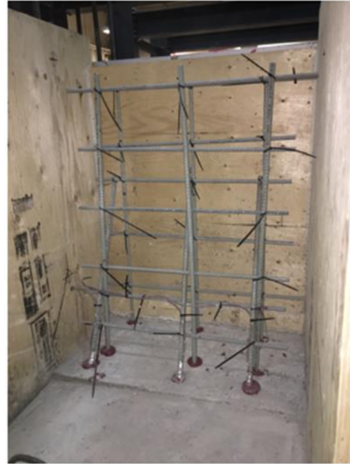
b) Post-installed wall prior to casting
