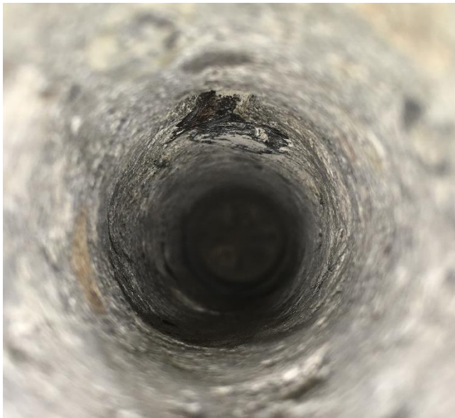
c) Inside of hole after cleaning
