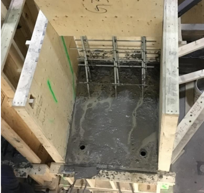
a) Pouring concrete over slab section
