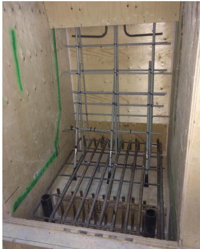
Figure 4.30: Barrier B-3 bar detailing prior to casting
