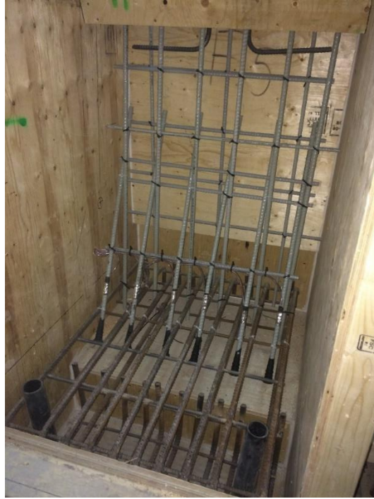
Figure 4.34: Barrier B-4 bar detailing prior to casting
