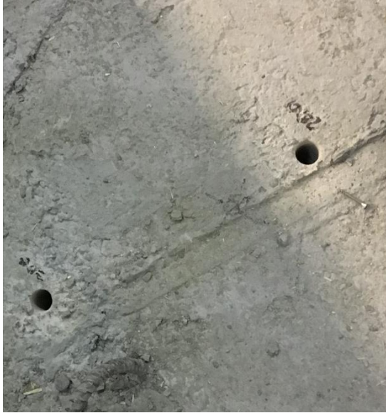
a) Post-Installed holes after drilling
