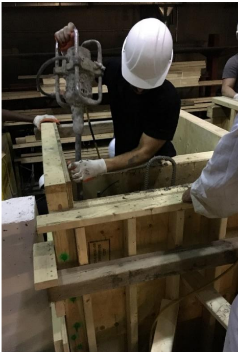
c) Vibrating poured concrete
