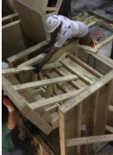
b) Lowering the timber side to cast the wall
