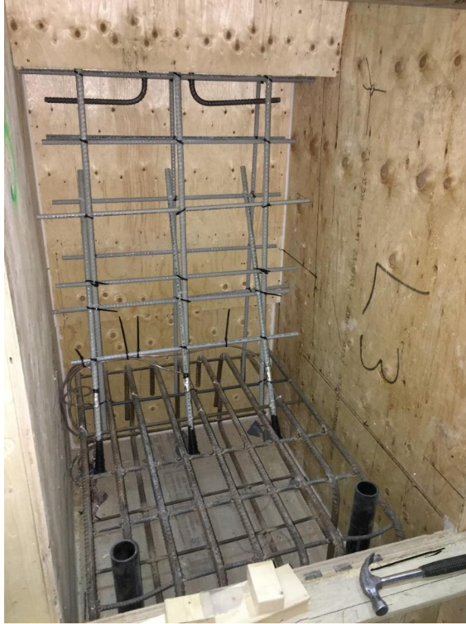
Figure 4.21: Barrier B-1 bar detailing prior to casting
