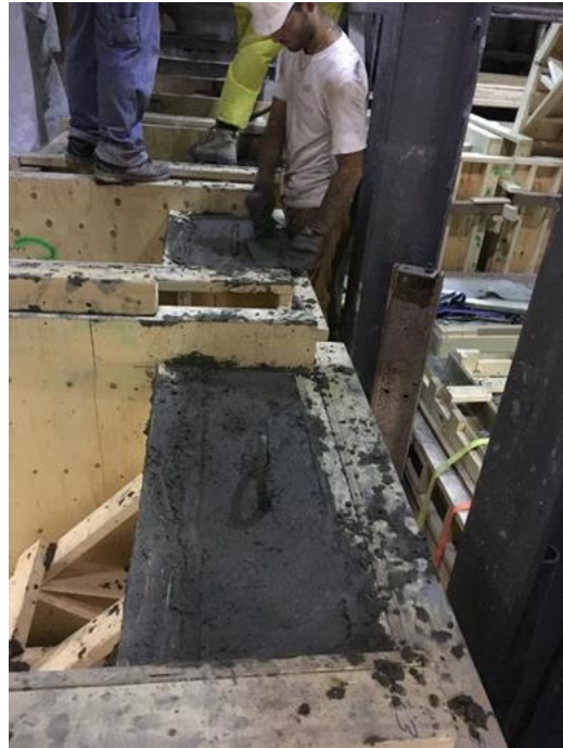
d) Smoothing concrete surface with a steel trowel
