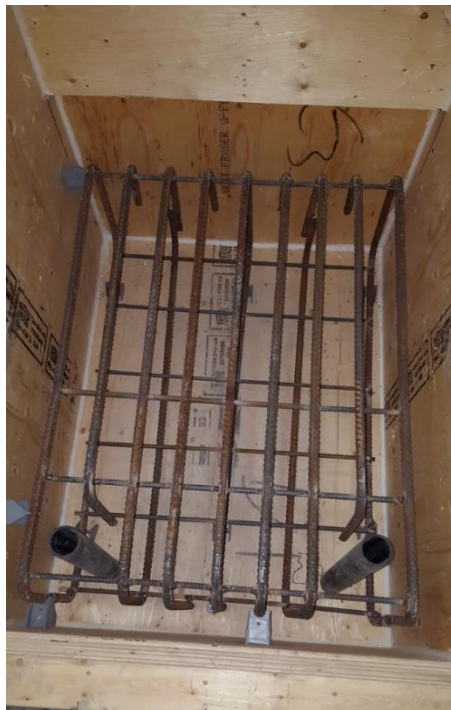
Figure 4.9: Slab steel reinforcement installation, and clear cover satisfaction
