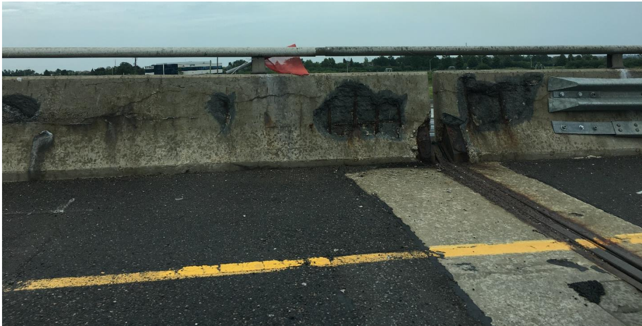
Figure 1.1: Photo of a deteriorated bridge barrier
