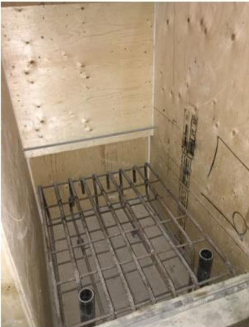
a) Slab prior to casting
