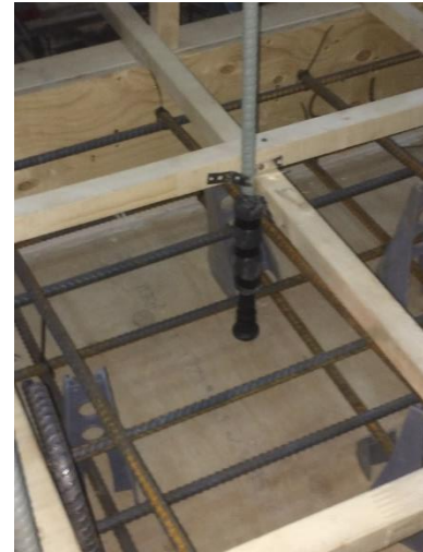
c) View of the headed bar with unbonded straight portion
