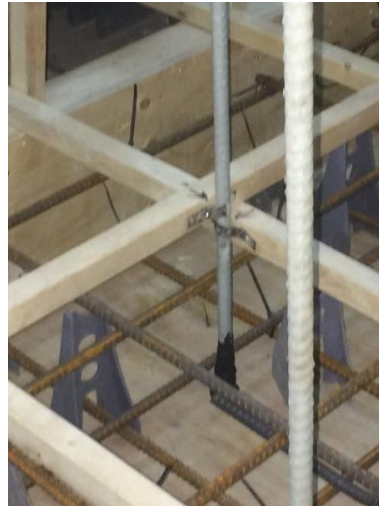
b) View of headed bar with fully-bonded embedment
