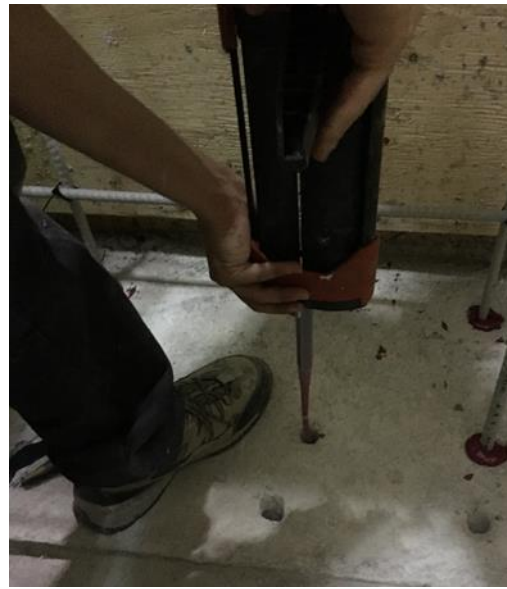
d) Injecting epoxy into drilled hole
