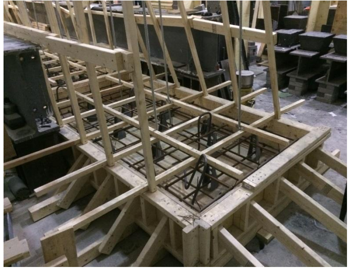
b) Transverse view of the timber form
