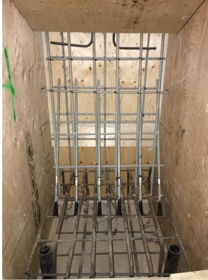
Figure 4.14: Typical GFRP wall mesh at exterior location
