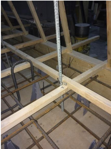
c) Close-up views of the bar with straight end
