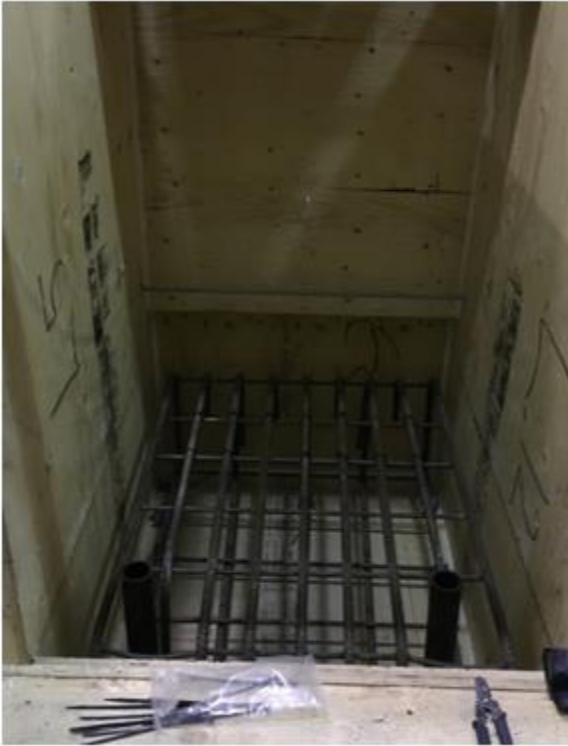
a) Slab reinforcement
