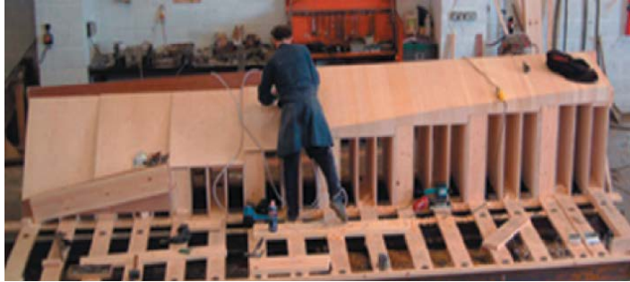
Figure 5.6.4.3 - 17 hand crafted timber formwork
