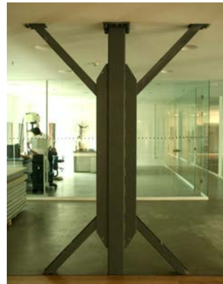
Figure 5.6.3.3 - Linear columns used in both planes act as truss
