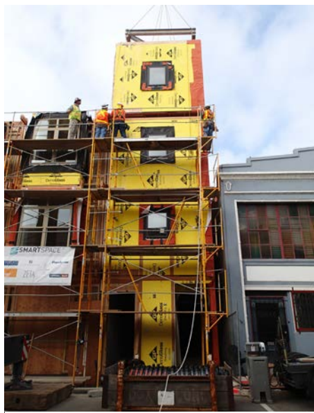
Figure 5.6.2.5 - Four floors of modules stacked in 4 days onsite
