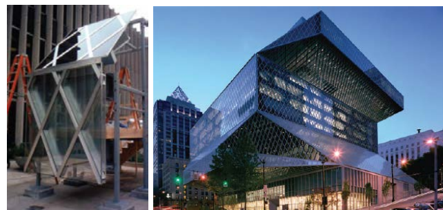
Figure 4.3 - Full-scale facade mock-up, Seattle Central Library
