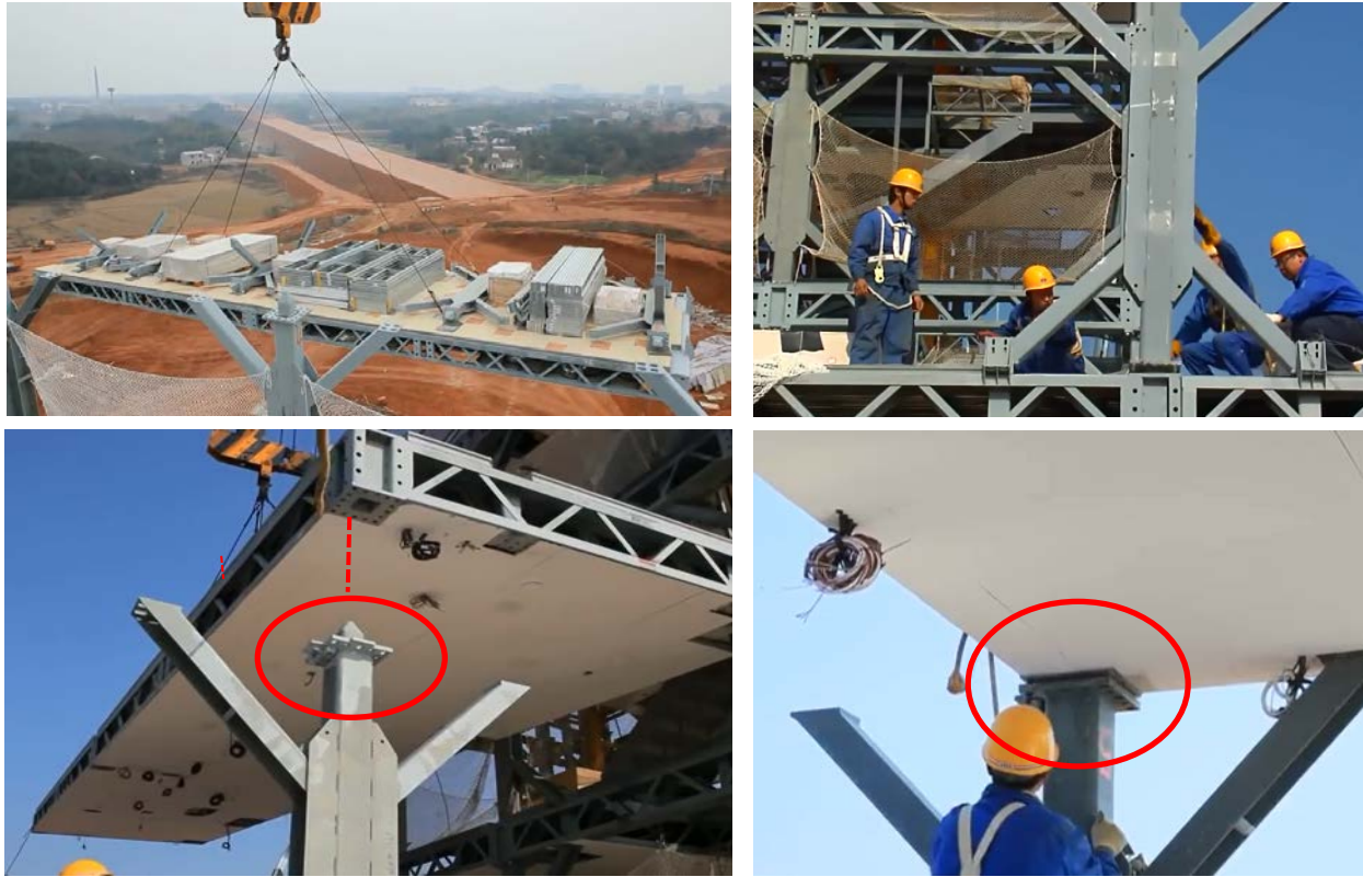
Figure 5.6.3.6 - Organized materials, vertical structure raised, floor mod set in place, and bolted together
