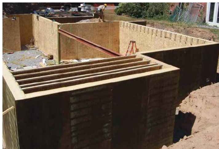
Figure 1.5. Views of the use of SIPs as preserved wood foundation in residential construction
