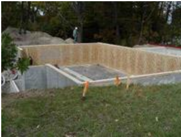
Figure 1.4. View of the proposed SIP foundation wall
