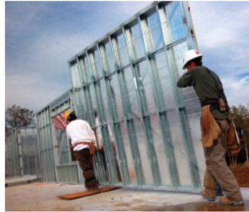
Figure 2.2. View of Lightweight Structural Cold-Formed Steel (CFS) ( http://www.steelframing.org )
