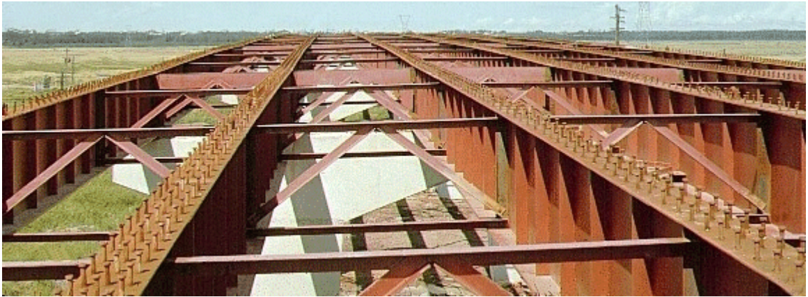
Fig. 2. 12. View of a steel girders in a bridge with shear studs
