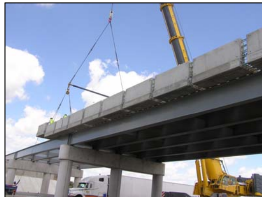
Fig. 1.2 Views of the Construction of Hwy 401/Mull Road Underpass Using Full-Depth, Full-Width, Precast Deck Panels with Reinforcing Steel (Source: MTO Bridge Office)
