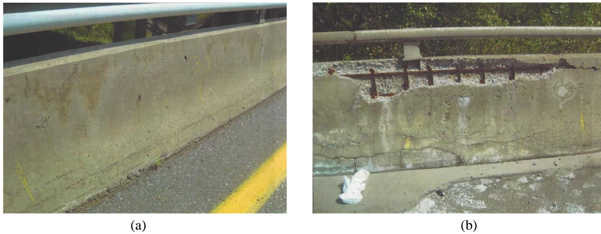
Figure 2.32: (a) Low deteriorated barrier at the East-North ramp, (b) High deteriorated barrier at the North-West ramp (Piersanti, 2015)
