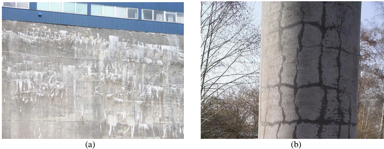
Figure 2.1: (a) Wall in Norway showing ASR gel extruding from the cracks (FHWA, 2008) (b) ASR damage on bridge pylon (Sika, 2013)
