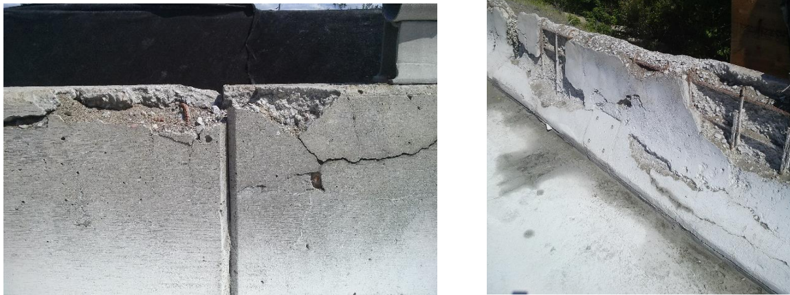
Figure 2.31: Signs of deterioration in highway bridge barriers (Piersanti, 2015)
