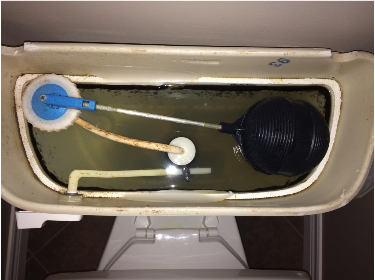
Figure 27: Toilet tank at House 9, with severe black mould buildup in the toilet tank.
