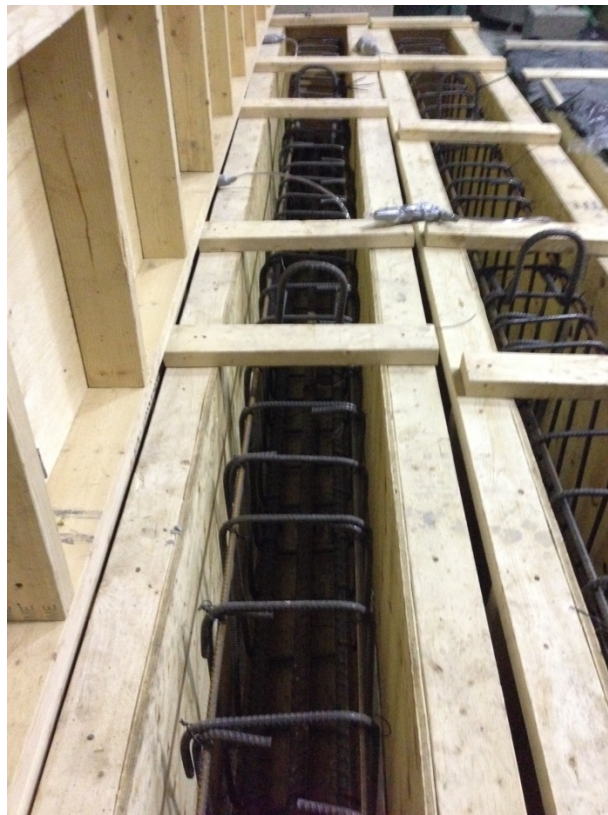
Figure 3.3.a – Manufacturing of HS-RC test beams - Formwork & rebar preparation
