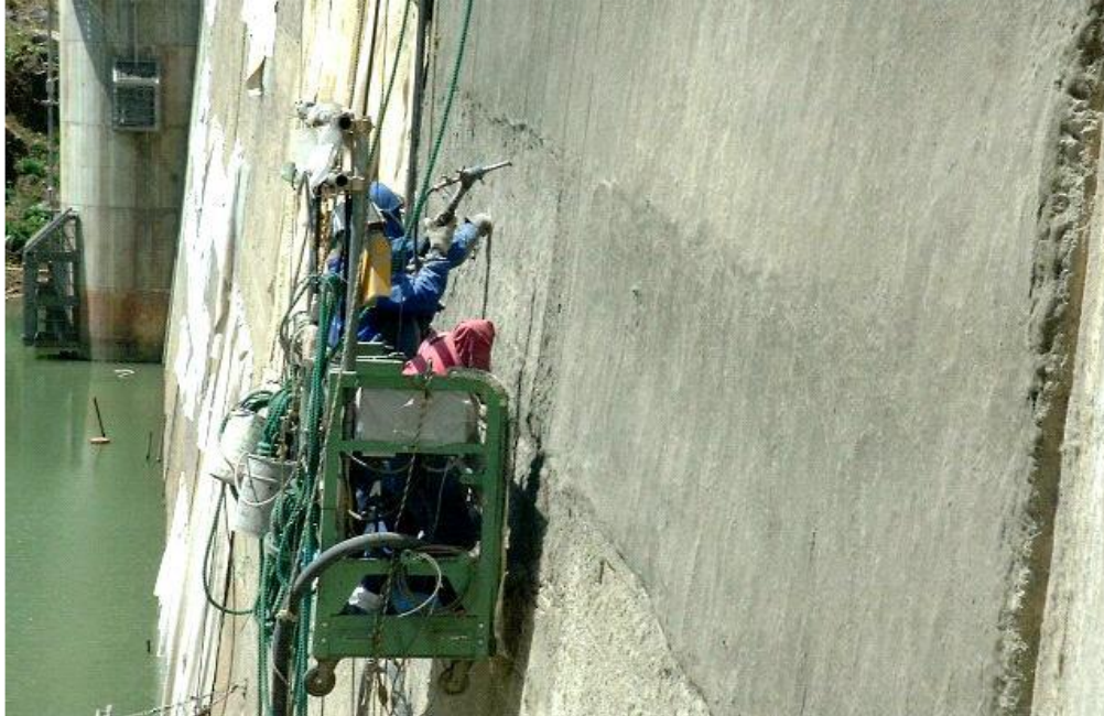
Figure 2.4 Spray repair of the Mitaka Dam with ECC for water-proofing (Kojima et al., 2004)
