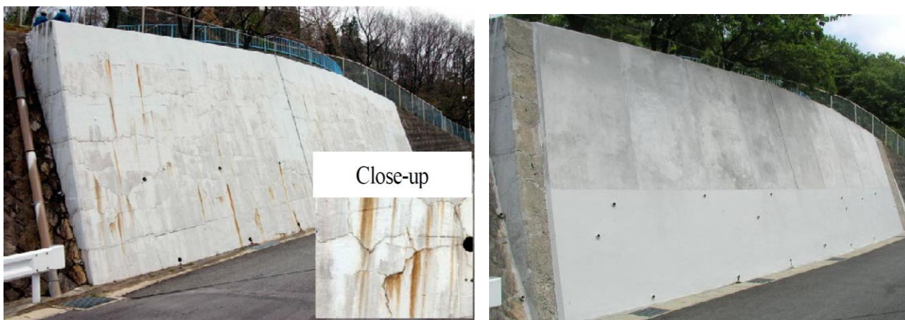
Figure 2.5: Surface repair of concrete retaining wall (Rokugo et al., 2005)
