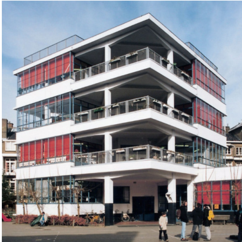
Figure 2.1: Open Air School in Amsterdam. After many renovations the classrooms, once open to the outside balconies, have been enclosed due to issues related to noise and mechanical HVAC.
