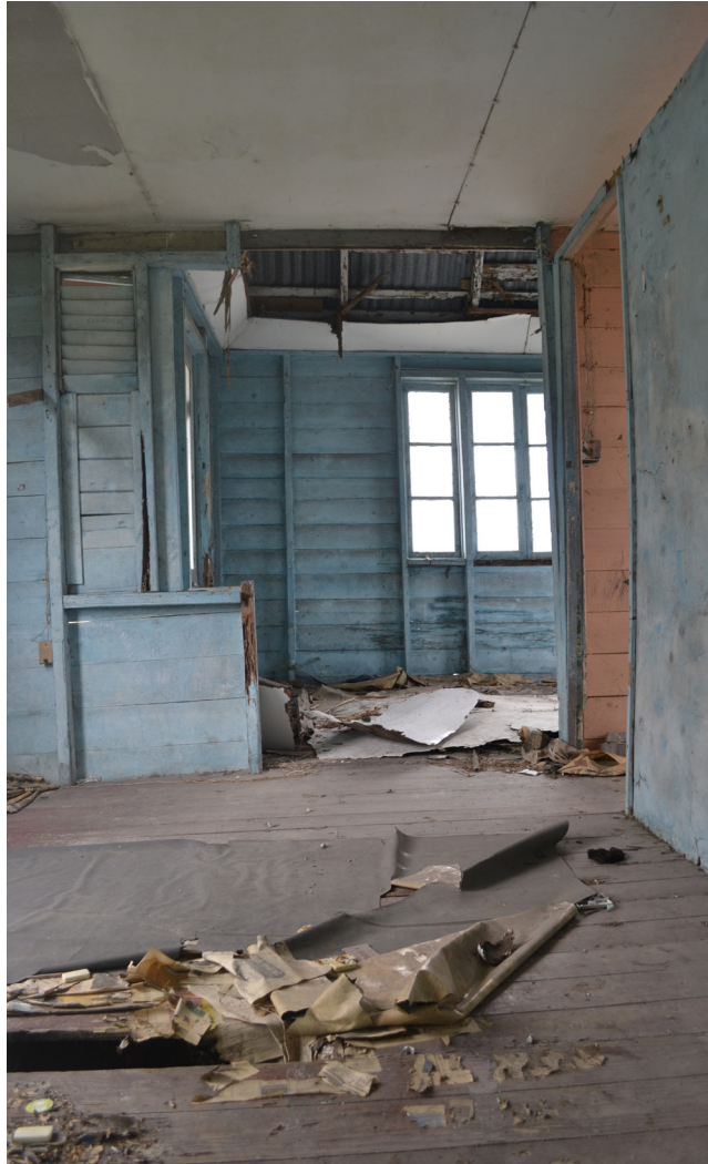
Figure 23: Interior Decay - standard spacing of timber studs was 2'-0".
