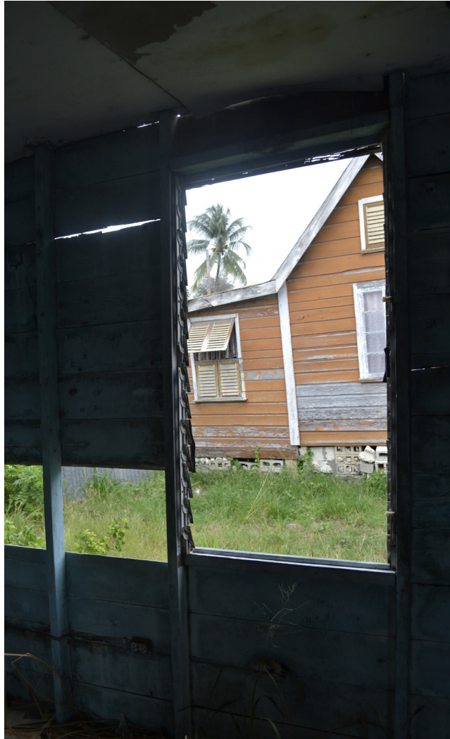
Figure 25: What's your story? Timber members spaced in accordance to the window and door openings.
