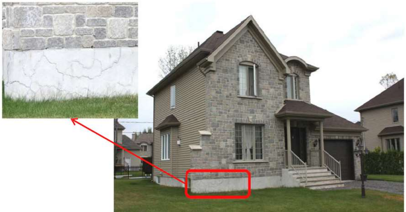
Figure 2.2. Deteriorations in concrete foundations (Rodrigues et al., 2012)
