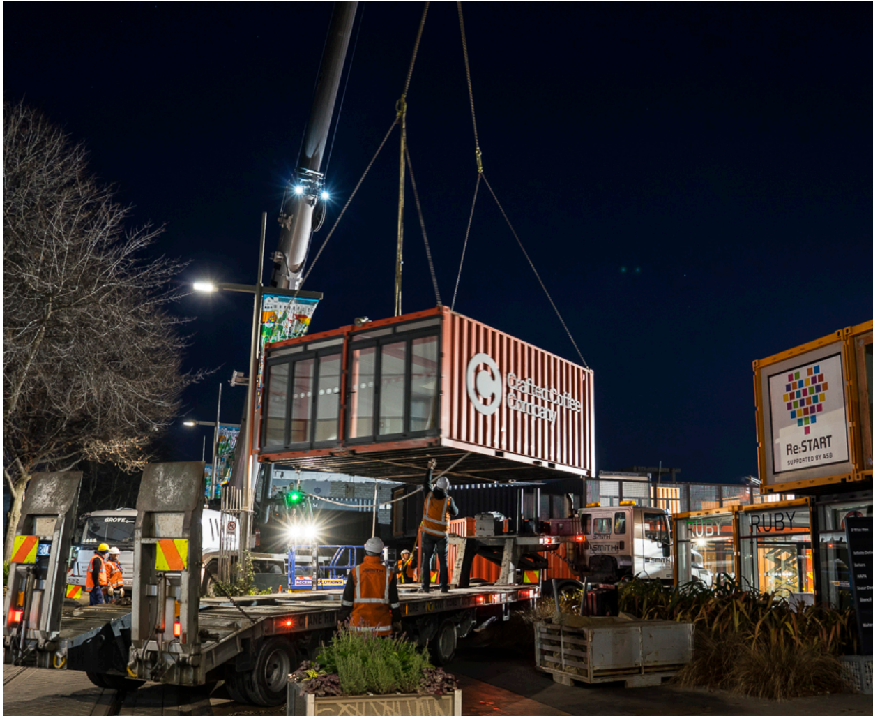
Figure 4. Modular construction with shipping containers. (Re:START, 2016)
