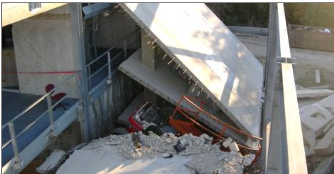
Figure 2.3.2: Collapsed building with floor sheet wedge between standing structure.
