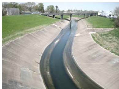
(a) Concrete ditches
