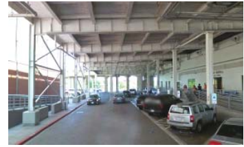
Fig 136(a). Underneath the Main St. Bridge. The University is built above the flood plain by resting on top of a parking garage that consists of a police station.
