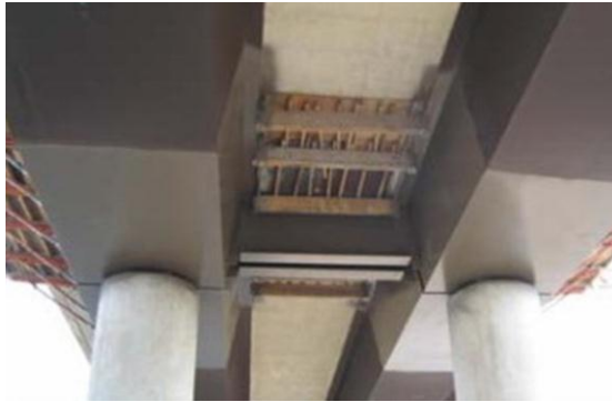
(a) Formwork at Soffit of Link Slab
