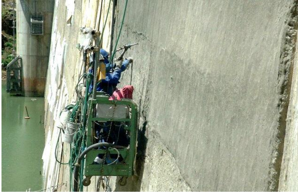
Figure 2.5 Spray repair of the Mitaka Dam with ECC for water-proofing (Kojima et al., 2004)
