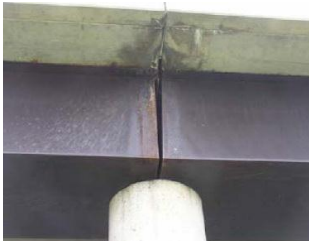
Figure 2.12 Typical Corrosion Damage Caused by Leaking Deck Joints (Lam et al., 2008)
