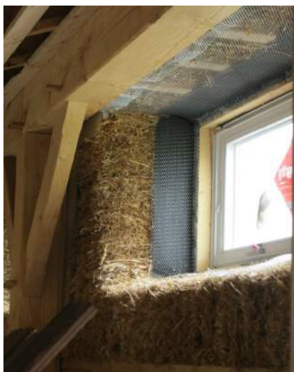
Figure 18: Tar paper/diamond lath air fin at window buck (Frey, 2014).
