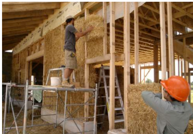
Figure 13: Double stud framing used with straw bale (Endeavour Centre).
