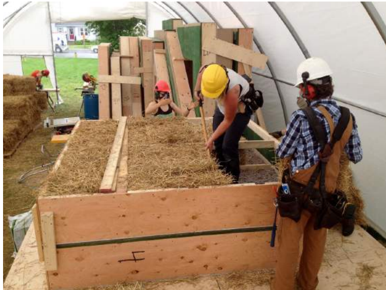
Figure 8: Straw SIP used in Zero House (Endeavour Centre, 2017).
