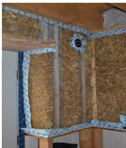
Figure 19: CONTEGA FC tape ready to accept stucco over straw bale (475 High Performance Building Supply, 2014).
