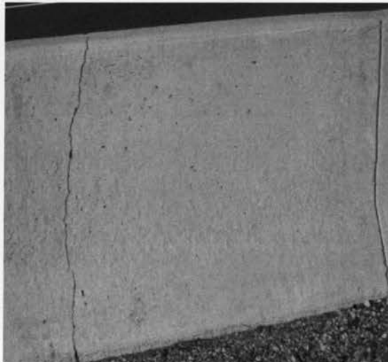
Figure 7.77: Photo of a plain concrete wall of approximately 3 years of age with vertical cracks
