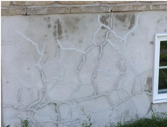
Map cracking in foundation
