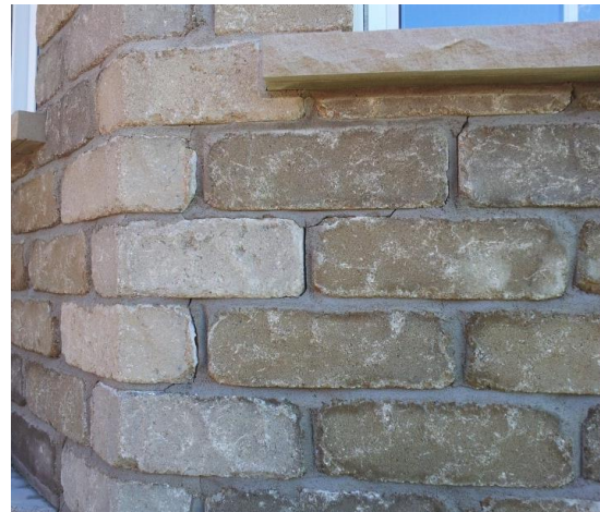
Cracked masonry caused by foundation expansion
