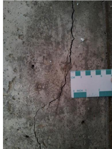
Interior crack in foundation
