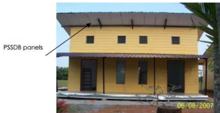
Figure 2.32 PSSDB roof panels (Awang & Badaruzzaman, 2010)
