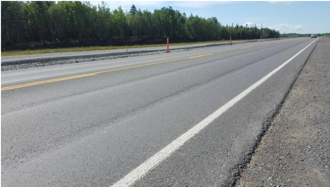
Figure 1.2: Parallel ruts on a highway (Source: https://www.cbc.ca/news/canada/newfoundland-labrador/worsening-ruts-government-experimenting-with-polymer-pavement-1.3196025 ).
