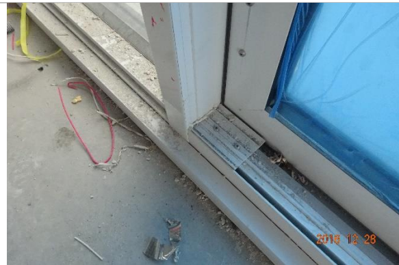
Door sill sash joint
