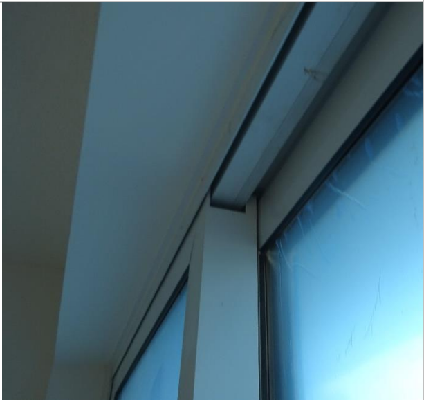
Door head frame and track
