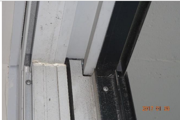
Fixed frame panel joint and weather stripping
