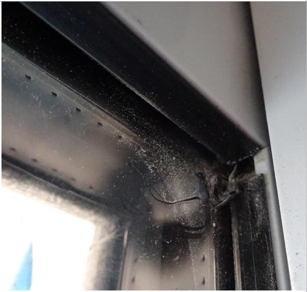
Sash corner joint
