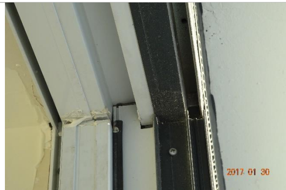
Fixed frame panel joint and weather stripping
