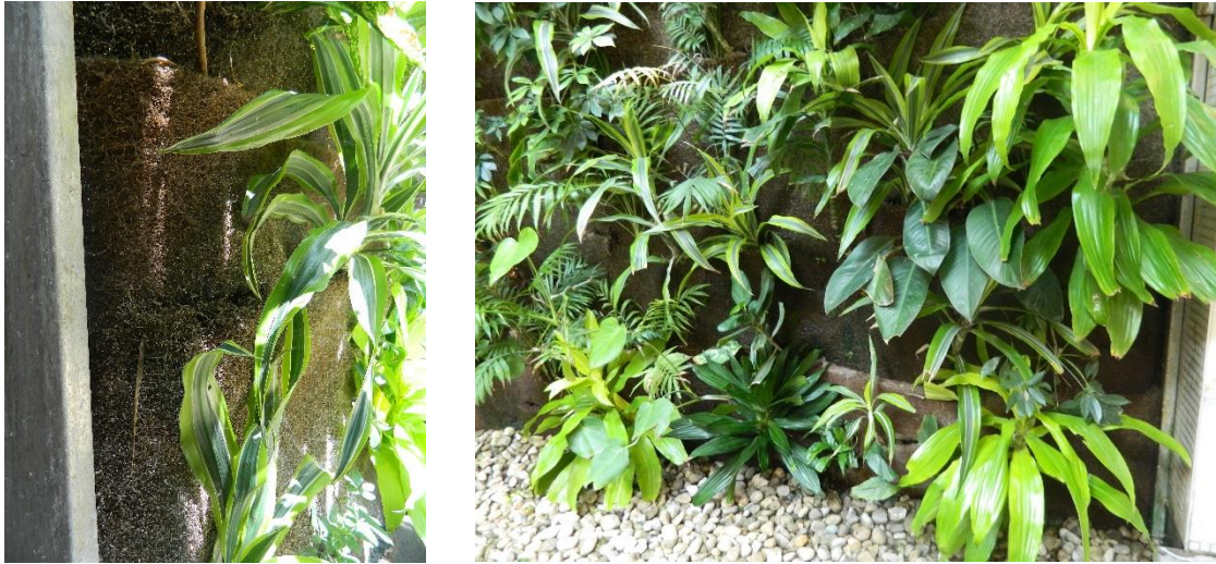
Figure 54: Living Wall investigated in this research, images showing the geotextile modules and the density of the vegetation
