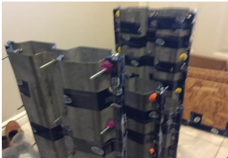
Figure 3.4 - Fabricated walls before casting
