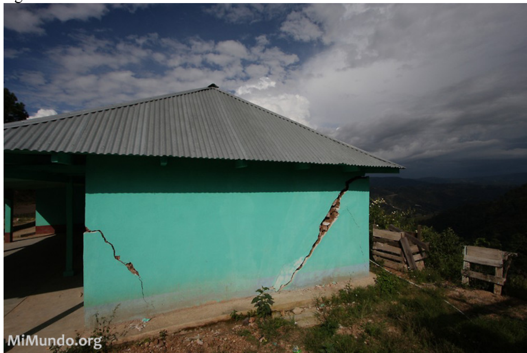
Owners of this home were forced to abandon it, as the cracks rendered it unsafe.
